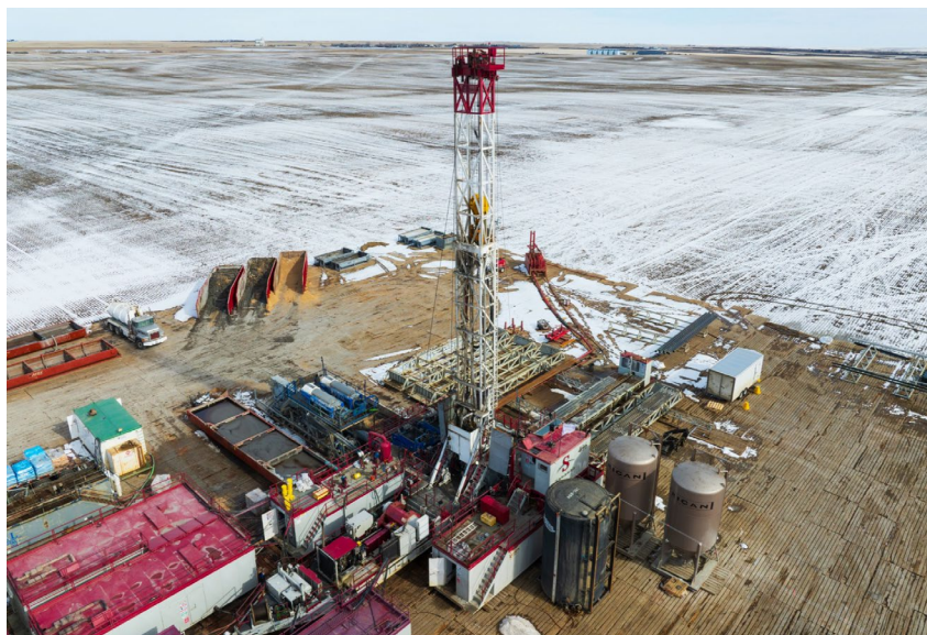
Drill rig at Bracken.
