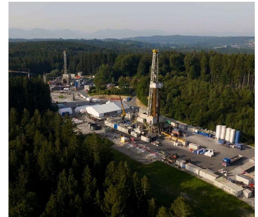
The Geretsried drill site.
