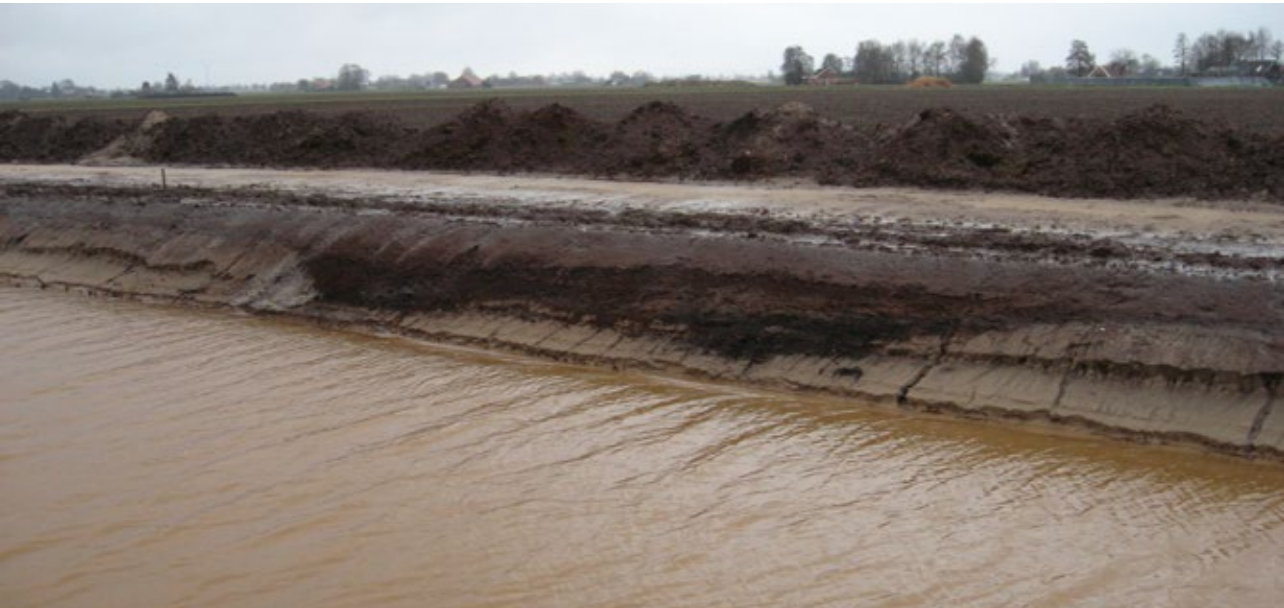
Example of an “unexpected” layer of peat whilst enlarging drainage channels in the Netherlands. This occurrence is very local and limited to a channel fill, but more extensive peat layers are common in coastal areas that experienced rapid post-glacial sea-level rise.
