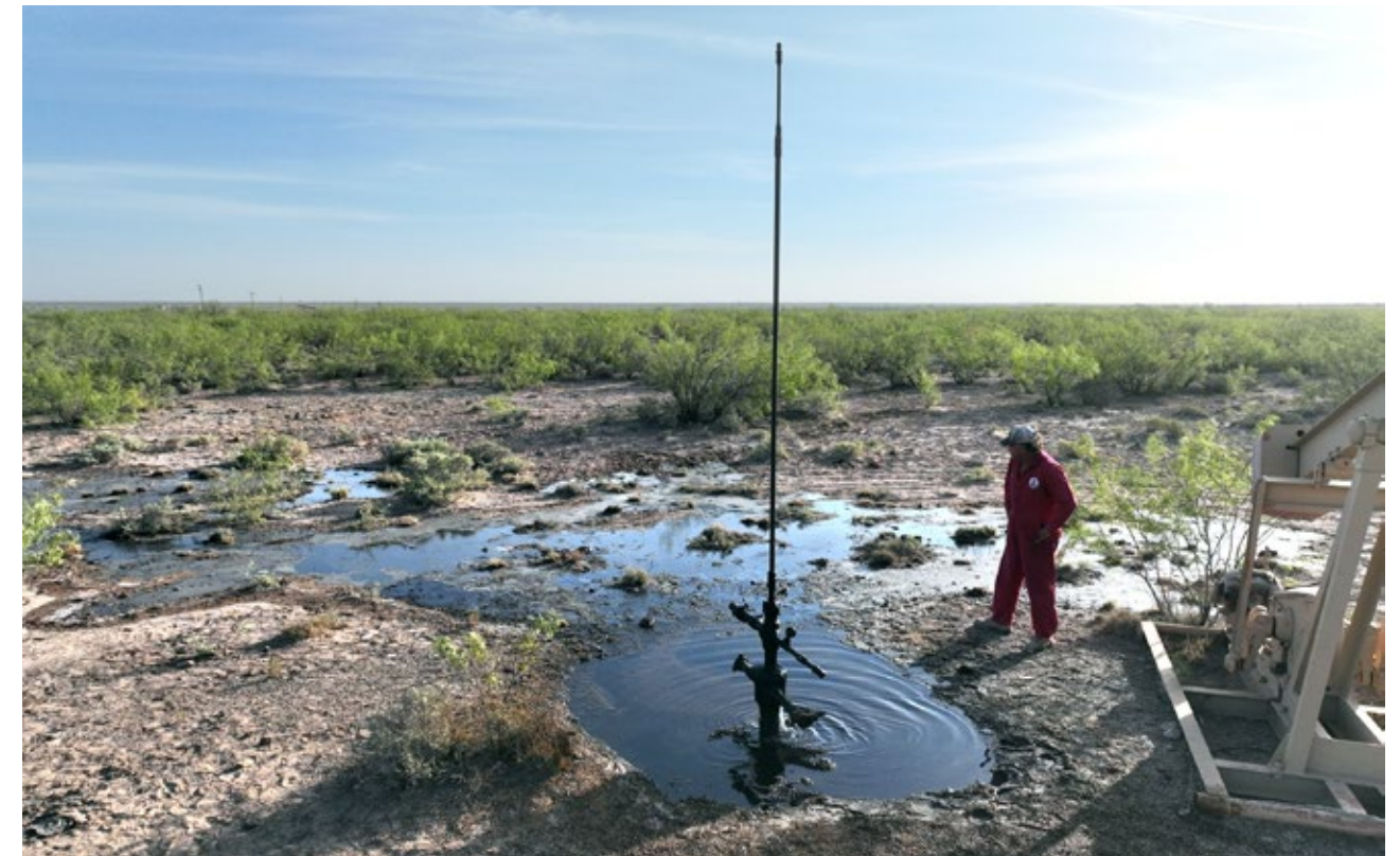
An orphaned well in Pecos that has catastrophically failed. Supported by the landowner, an investigation was carried out to assess where flow was coming from.
