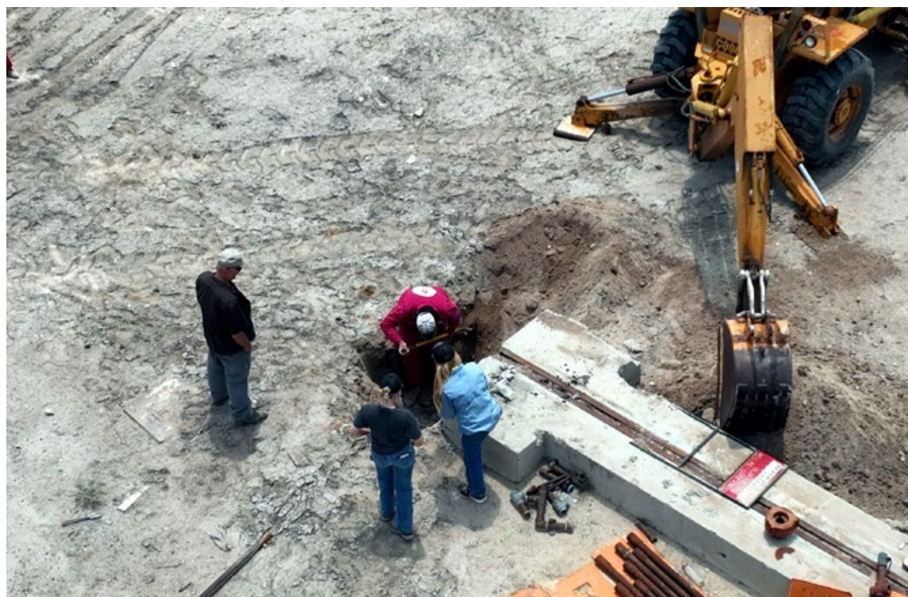
An orphaned well in Pecos that was "plugged" by an RRC contractor about two years ago. It was excavated in July 2024 and confirmed that it is leaking water and volatile organic compounds.
