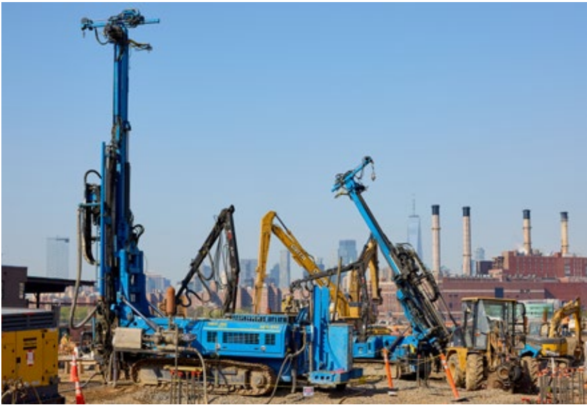
Geosource Energy rigs on Java Street, Brooklyn, New York. This 321-borehole project is the largest geothermal residential development in New York State.
