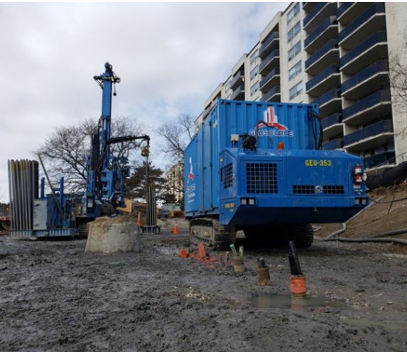
The 240 Markland project, Toronto, Canada, is a retrofit of a 10-storey multi-residential building with angled boreholes. See how tight some of these boreholes are at surface.
