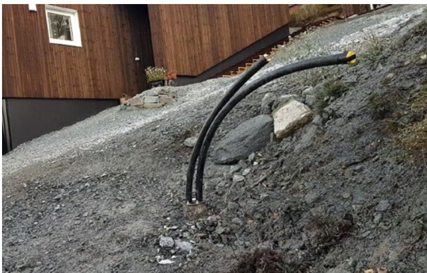
The two connected tubes of a closed geothermal loop drilled in 2017 in Trøndelag. Antifreeze is circulated through the tubes to utilize the heat at a depth of up to 200 metres.
