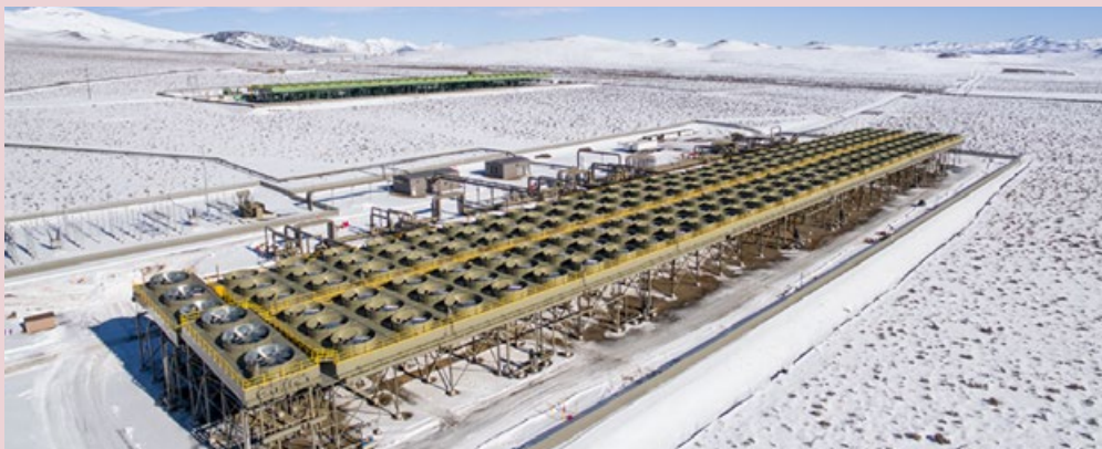
McGinness Hills is the largest pumped-well geothermal plant in the world. As of 2021, the installed capacity at McGinness Hills is estimated between 150-170 MWe (gross).
