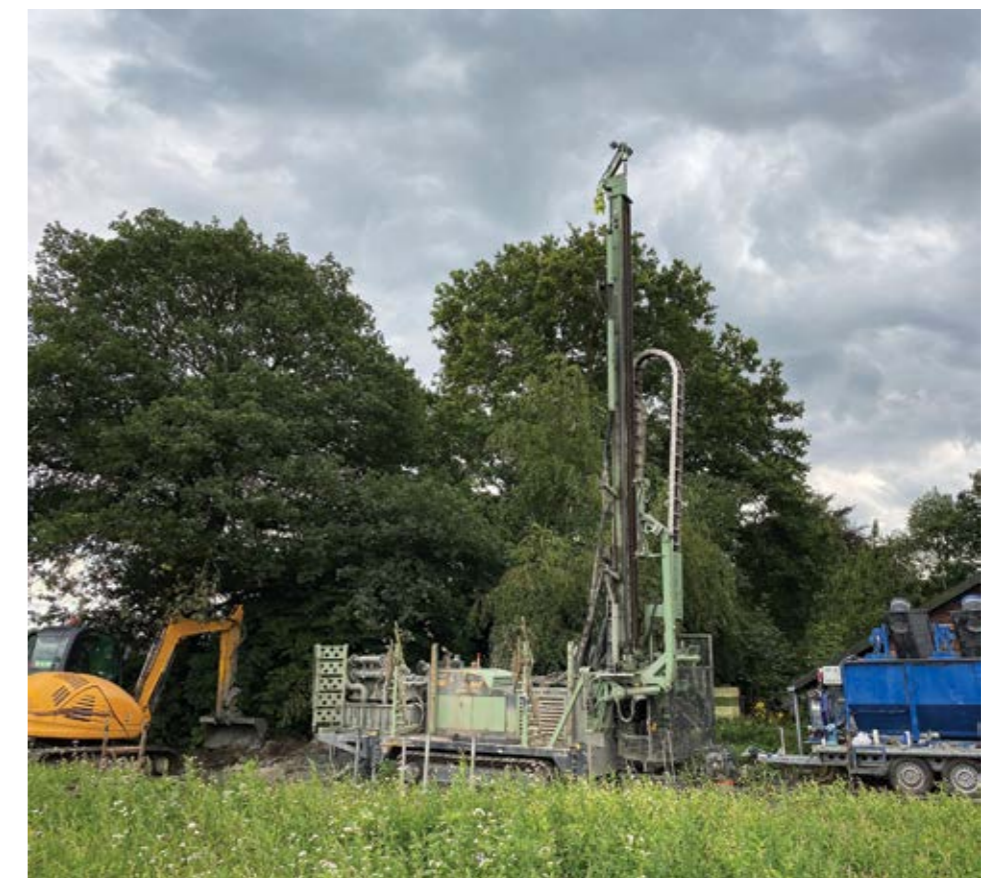
Drilling ongoing in Jan Rossingh's back yard.
