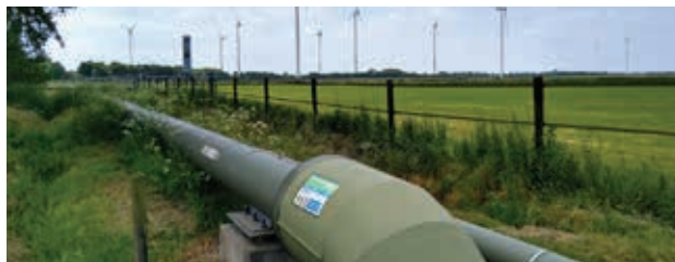
New pipelines of the NAM Schoonebeek redevelopment in the Netherlands against a backdrop of a typical landscape that is characterised by farmland and wind turbines.
