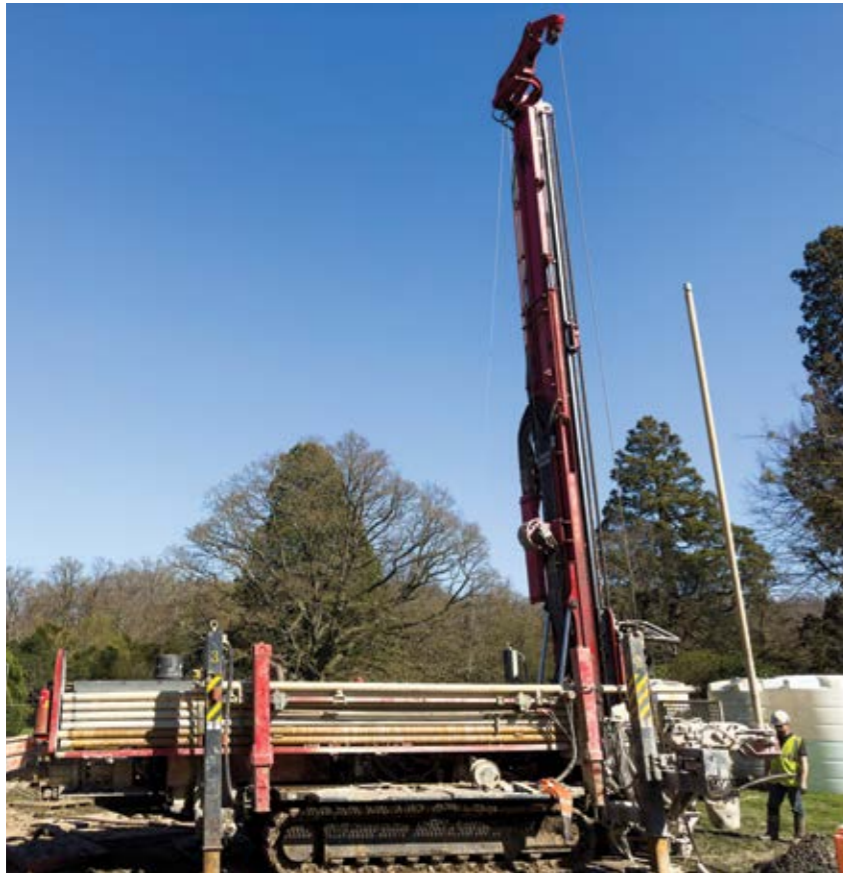
One of GTD’s drilling rigs in action.
