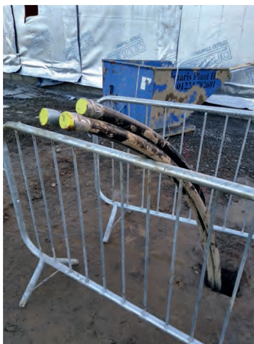
An impression from the drill site once the tubes have been placed in the borehole.
