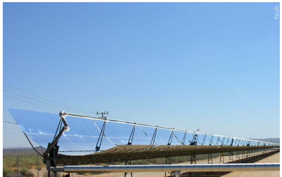
This is a parabolic trough solar thermal electric power plant in California. According to IEA, the use of renewable energy will triple between 2008 and 2035, driven by the power sector, where their share in electricity supply rises from 19% in 2008 to 32% in 2035.
